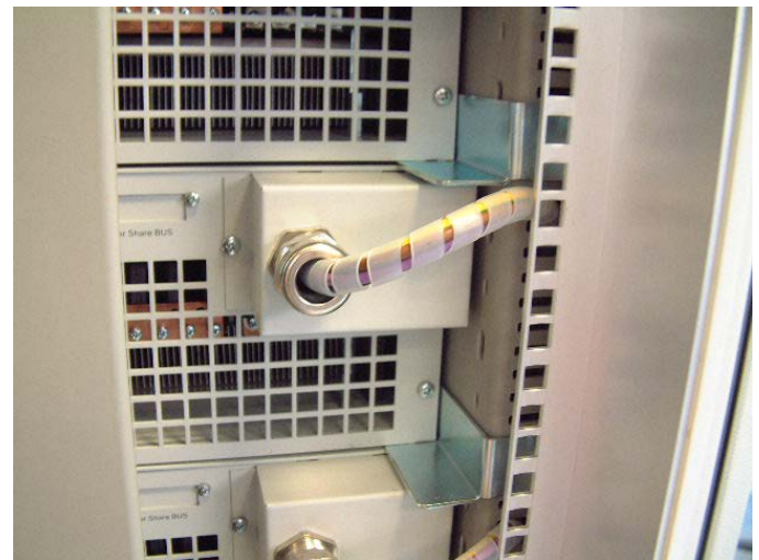
Figure 1: AC input connection of the single units
