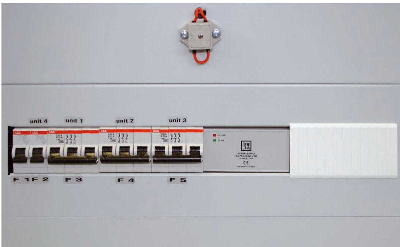
Figure 8. Front with input breakers and external emergency off contact
