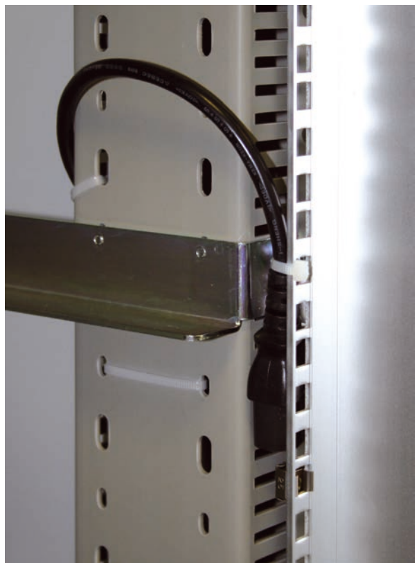
Figure 6. Spare AC power connector for load
