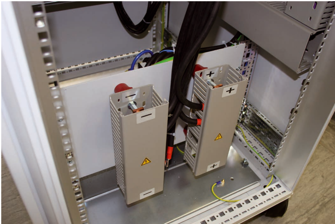
Figure 7. Covered DC connection terminal
