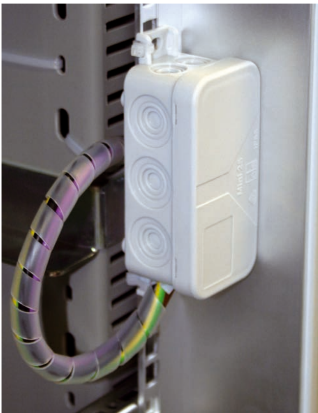
Figure 5. Spare AC input cables for power supply
