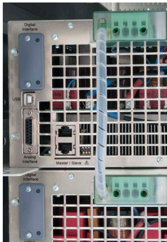
Share-Bus-Verdrahtung (Systeme 1 und 2) / Share bus wiring of systems 1 and 2
