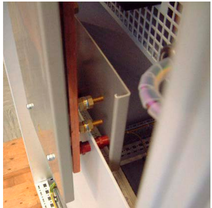
Figure 4: DC output terminals
