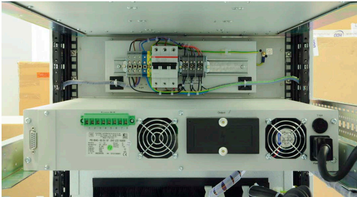
Figure 7 - Rear view of power supply unit and ENS2 unit
