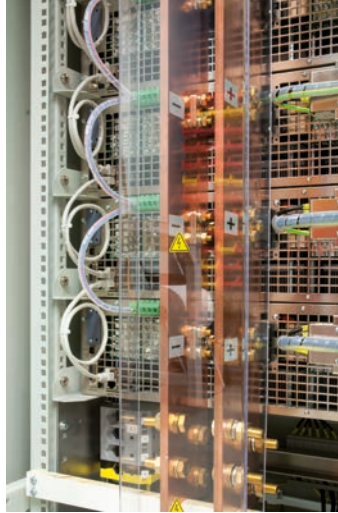
Bornier bus DC / DC bus terminal
